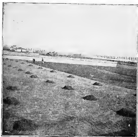
CLEANING A FILTER, EAST LONDON.
